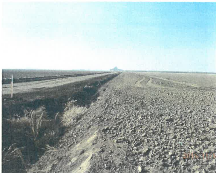
Dixon RCD Lateral 4a: Site preparation Nov. 2015
