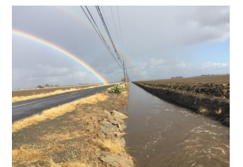
Tremont 3 at Hackman Road October 25, 2021
