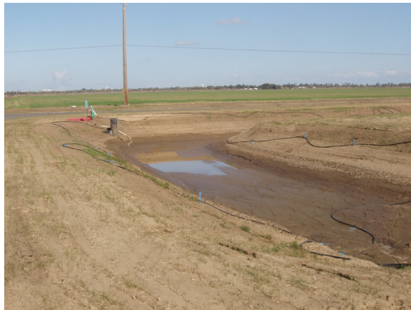
Timothy Sediment Basin at Runge & Tremont Roads Post-Oct. Storm. Will control sediment from two 30 acre fields. NRCS Photo
