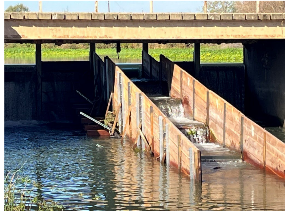
Recently SCWA staff worked with the farmers and CA Dept. of Fish & Wildlife to install a temporary Fish Ladder to a water control structure, allowing flooding of habitat on the Yolo Bypass Wildlife Area and fish passage to happen simultaneously
