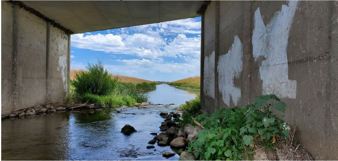
Figure A.34. The view looking downstream at Ulatis Creek.
