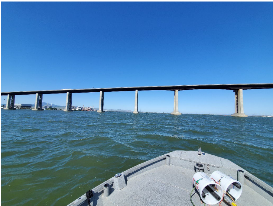
Figure A.23. Site CONF-010 on the San Joaquin River just upstream of the Antioch Bridge.
