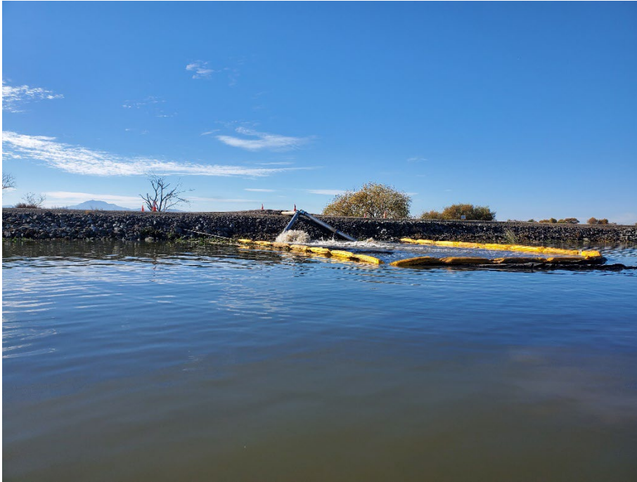
Figure A.4. Water from a channel dredging operation being pumped into the San Joaquin River.
